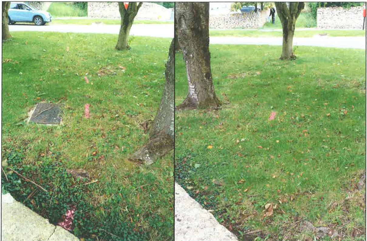
Figure 28 – SSE Survey 27 Aug 2020 (29 cable / [REDACTED] Cable)
